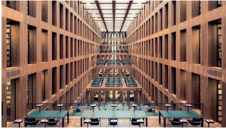
Figure 28 – Jacob and Wilhelm Grimm Centre, symmetric framed shot exploring the building grid lines (image source: Stewart 2016).
